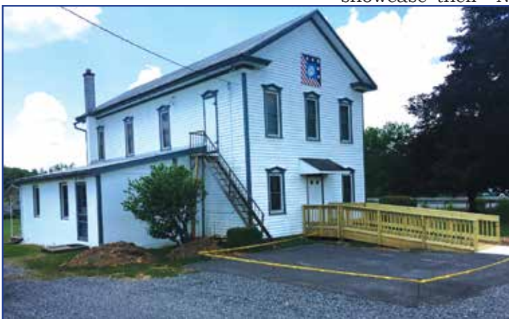
(July 2020) The new and improved entrance to the historic Eagle Grange Hall; note the accessible ramp and the reserved handicap parking area. (Photo Credit: David Troutman)
